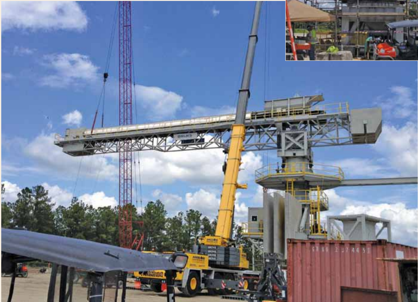
Setting of a large stacker
