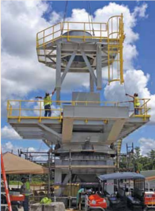
Alex Mercado and Harold Peters setting a section of a stacker conveyor
