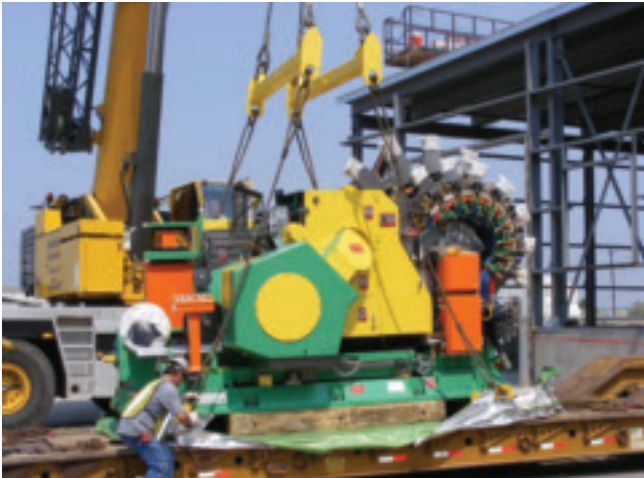
At the Ball Corporation project in Ft. Worth, members used an 8-color decorator weighing 56,000 pounds
