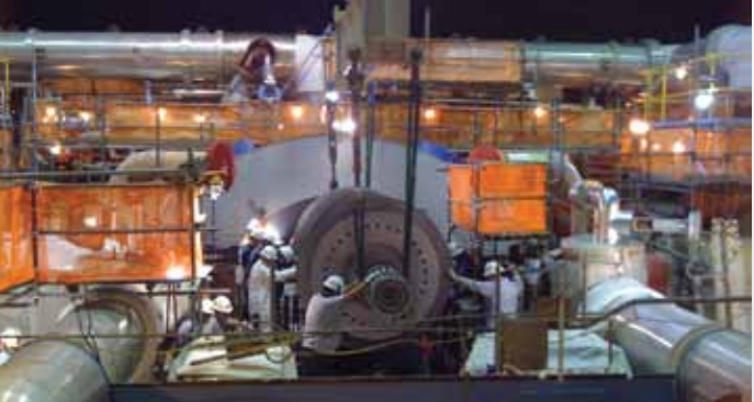
Siemens rigging in a turbine rotor at Turkey Point Nuclear Plant in South Florida
