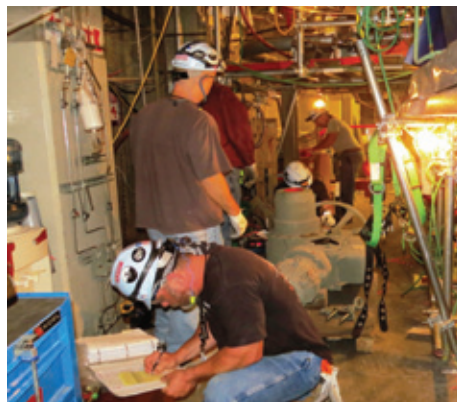
Chad Snow, Edwin Miller, Sam Everhart, Billy Smithwick, and Jamie Donald install a motorized valve operator. This is considered to be a complexed lift while rigging it into place. The weight of the machinery is about 2,300 pounds.
