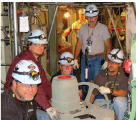
Chad Snow, Edwin Miller, Sam Everhart, Billy Smithwick, and Jamie Donald install a motorized valve operator. This is considered to be a complexed lift while rigging it into place. The weight of the machinery is about 2,300 pounds.
